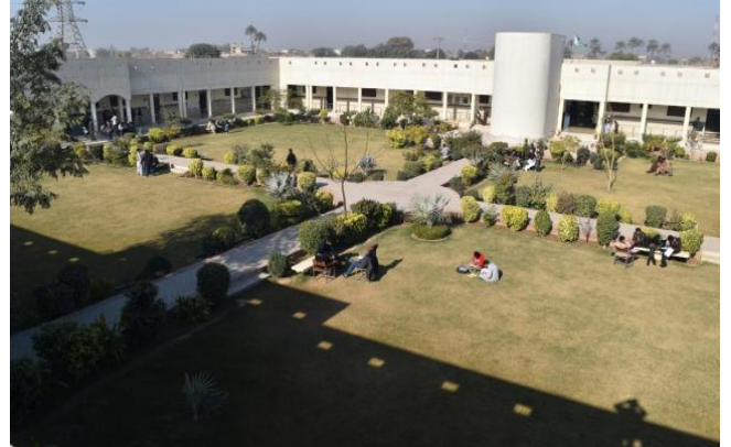
Lawns inside the Building (Post Graduate Block)
