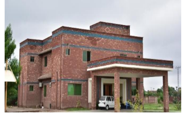
Building in Block B (Guest House) Area 611 m 2
