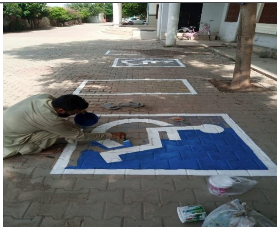
Repainting of Parking Signs
